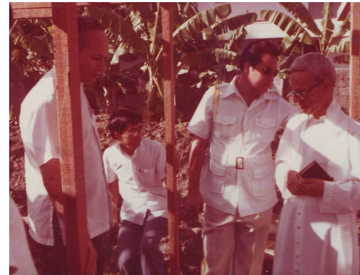
On the site of on-going seminary construction, with Fr. Antonio Barbangelo, 1980
